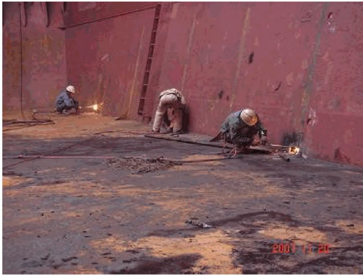
Photograph 1 Heavy corrosion affecting inner bottom plating
