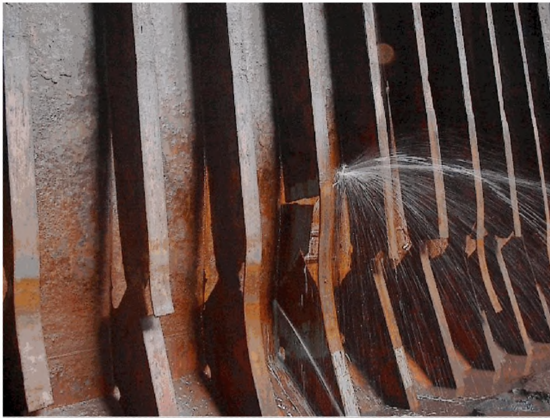
Photograph 1 Leakage from side shell plating due to heavy corrosion
