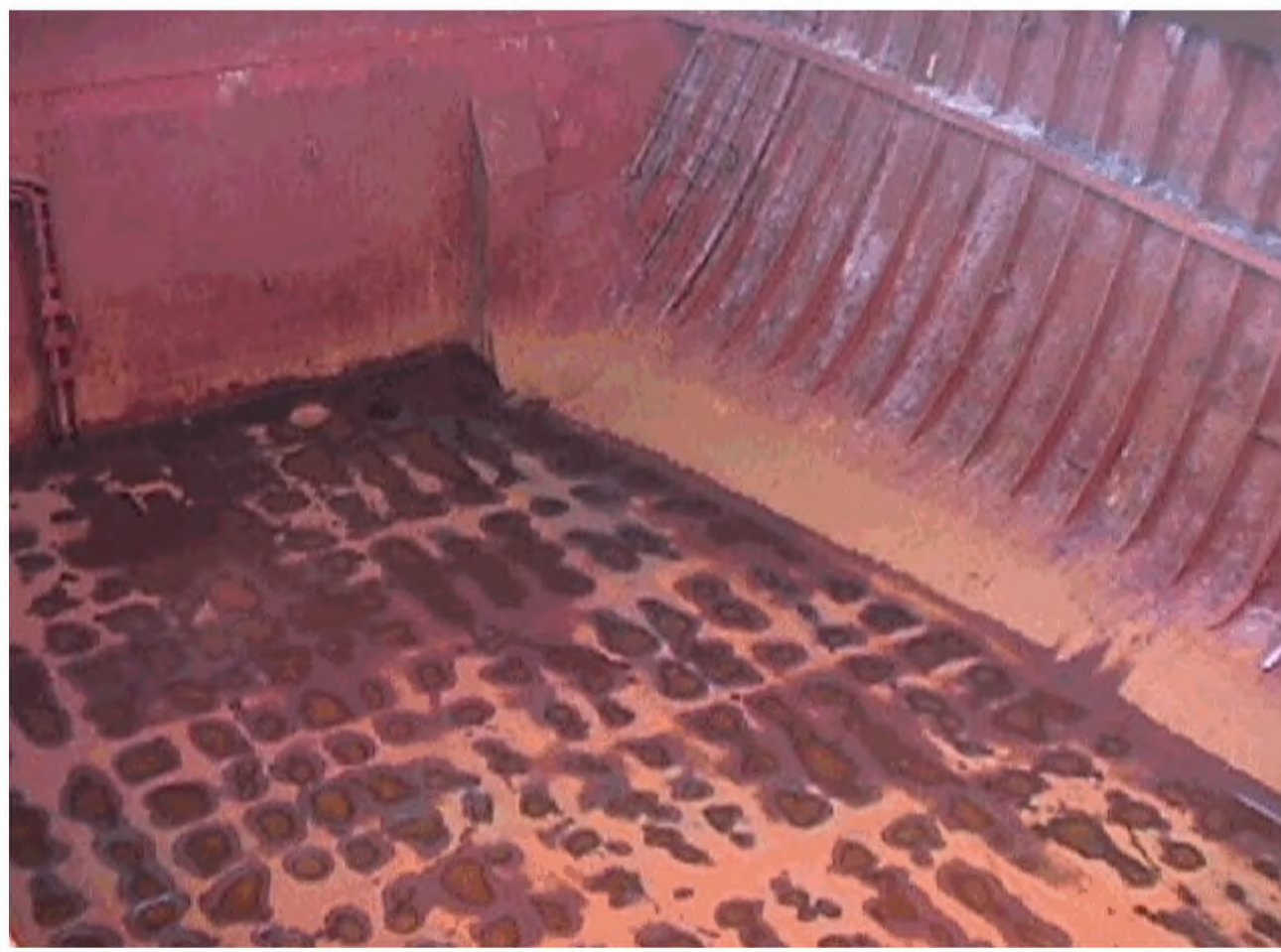
Photograph 2 Damaged inner bottom plating
