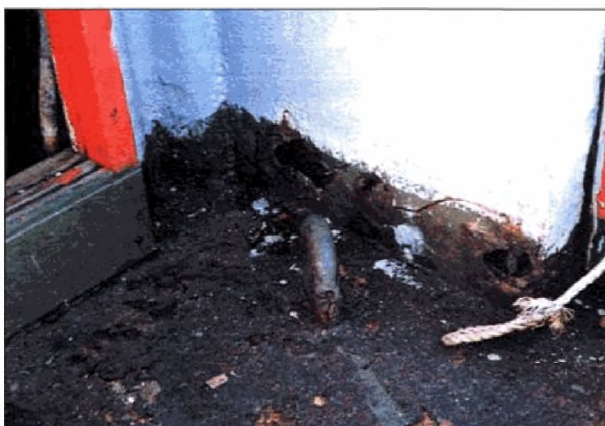
Photograph 1 Corroded accommodation house side structure
