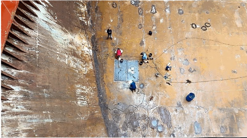
Photograph 3 Repairs of damaged inner bottom plating
