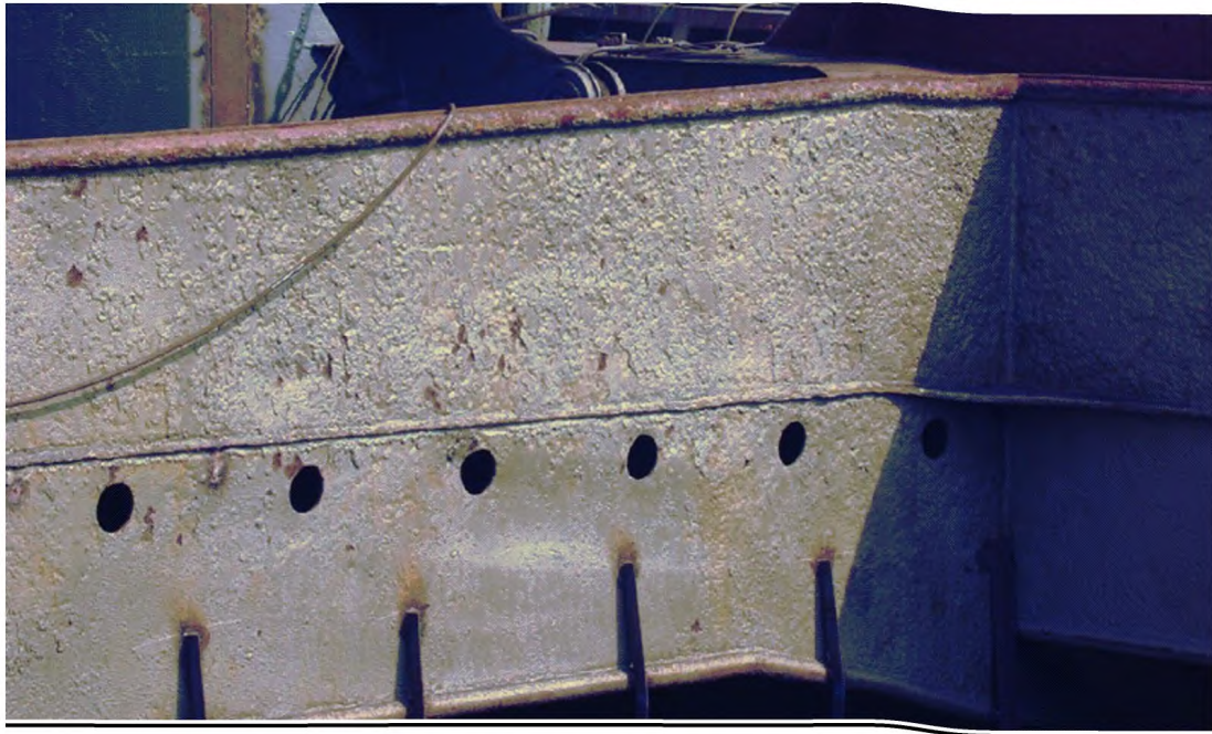
Photograph 1 Heavy corrosion of hatch coaming
