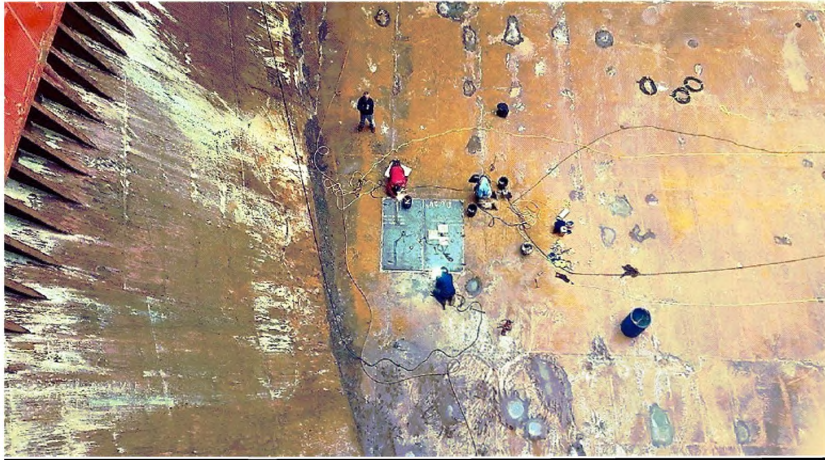
Photograph 3 Repairs of damaged inner bottom plating
