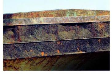
Photograph 1 Heavy corrosion of hatch coaming and topside tank plating vertical strake
