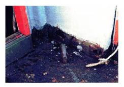
Photograph 1 Corroded accommodation house side structure
