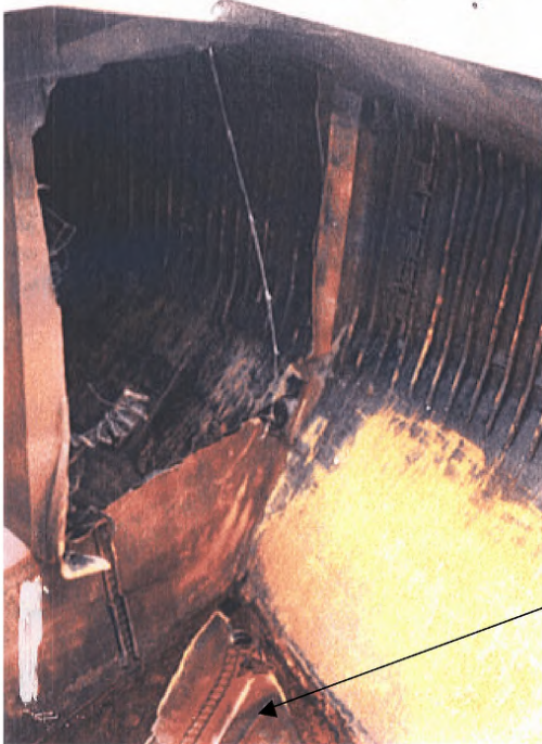
Photograph 1 Collapsed and detached transverse bulkhead
