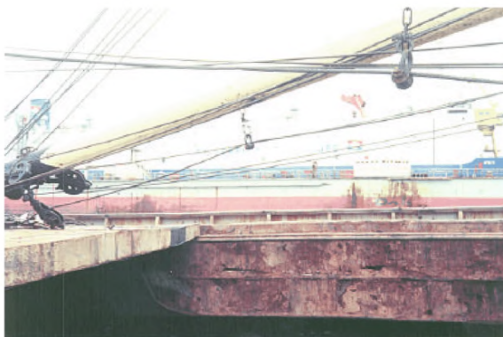
Photograph 1 Heavy corrosion of hatch coaming
